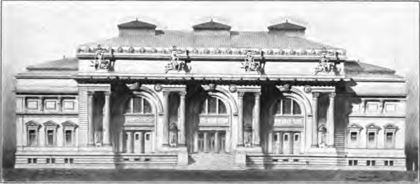
THE NEW WING.
